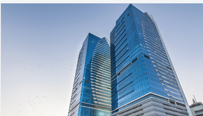
Sky Towers (East & West Wing)
